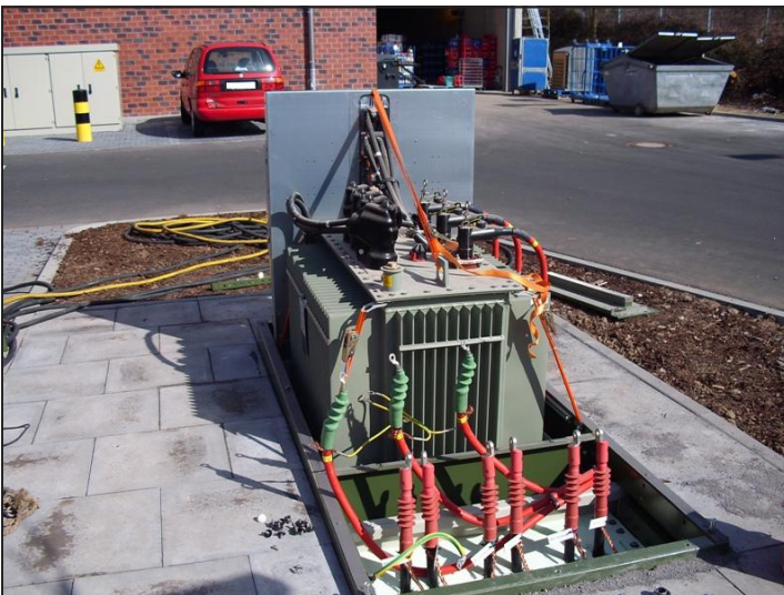
LCS-E, housing detached on-site
