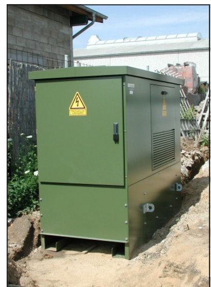
positioned LCS-E without basement
